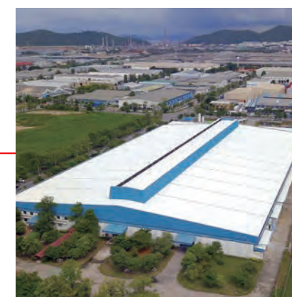
Fujitsu General (Thailand) Co., Ltd. (Thailand) Factory-2
