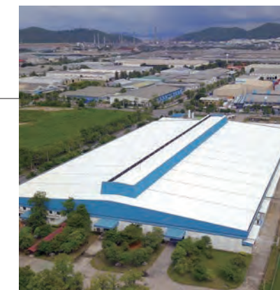
Fujitsu General (Thailand) Co., Ltd. (Thailand) Factory-2
